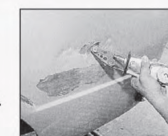
Paint removal work on concave surfaces
